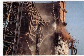
A wrecking ball is dropped through the upper portion of the coal pulverizer building, sending a shower of debris to the ground below.
